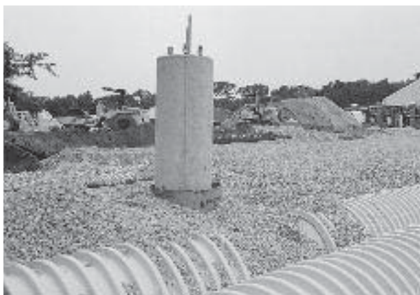
Figure 15 – Chamber bed placed around light post.
